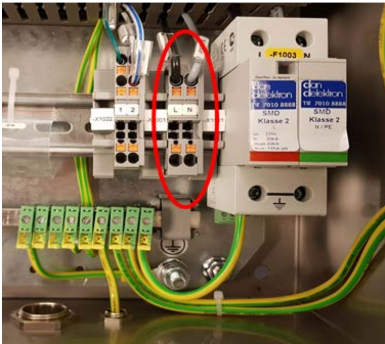
Figure 43 - READY Collector Base mains connection
