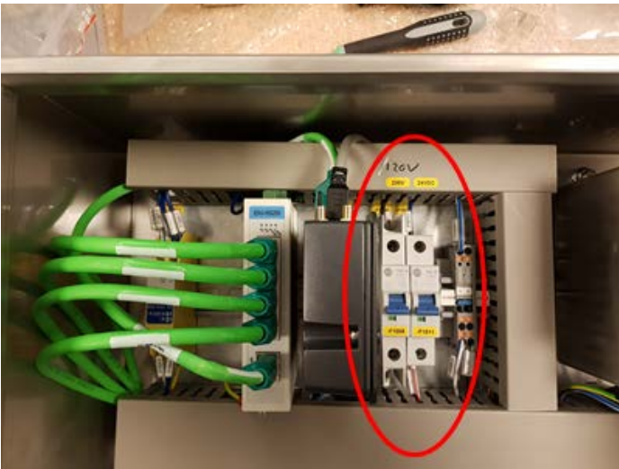
Figure 44 - REAdy Collector Base 120/230 VAC & 24 VDC power switches
