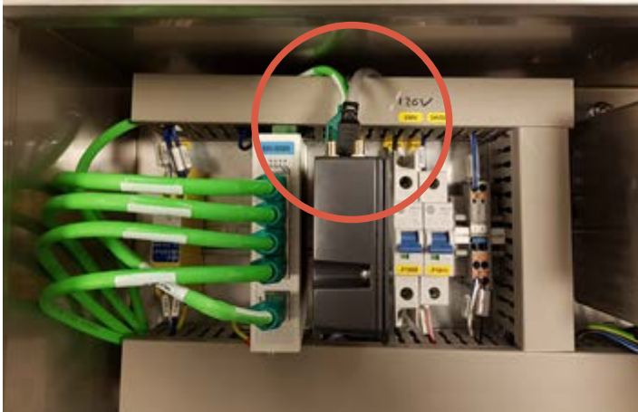
Figure 38 - LAN and power connection, SIERRA Wireless RV50x
