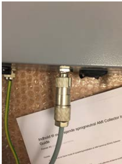
Figure 27 - Power connection installation 2
