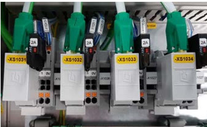
Figure 33 - READy Collector Base 24VDC connection
