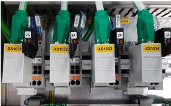
Figure 32 - READy Collector Base Ethernet connectors
