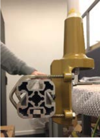
Figure 24 - Antenna installation on antenna beam
