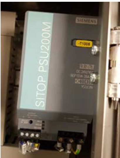
Figure 42 - READy Collector Base power supply
