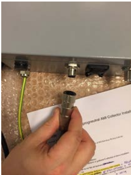
Figure 26 - Power connection installation 1
