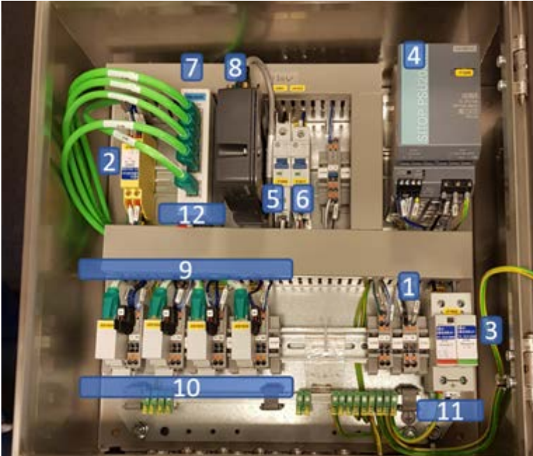
Figure 5 - READy Collector Base inside view
